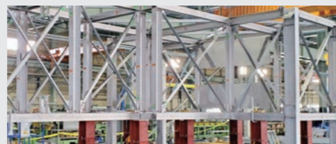
Example of stainless steel building structure engineering
