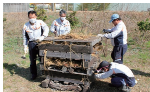
Creating and installing an "insect hotel" habitat for insects in Nakashinden green spaces as part of biodiversity preservation initiatives
