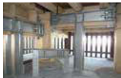
Seismic strengthening works of a five-story pagoda
