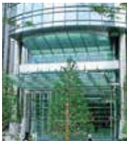
Entrance eave, curtain wall
