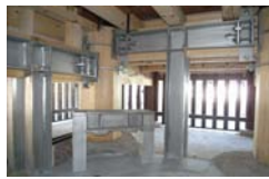
Seismic strengthening works of a five-story pagoda
