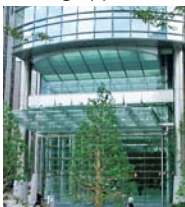
Entrance eave, curtain wall
